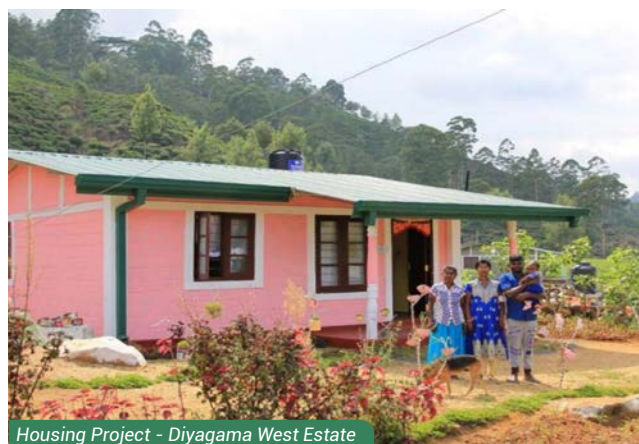
Housing Project - Diyagama West Estate
